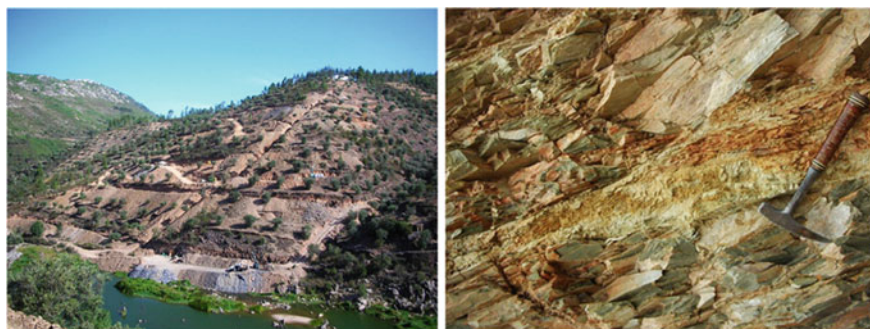
Fig. 5 Trenches excavated to investigate a dam site (Portugal) ( left ) and a detail of a fault containing clay gouge observed in a trench wall ( right )
